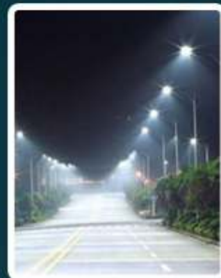
LED STREET LIGHTS
